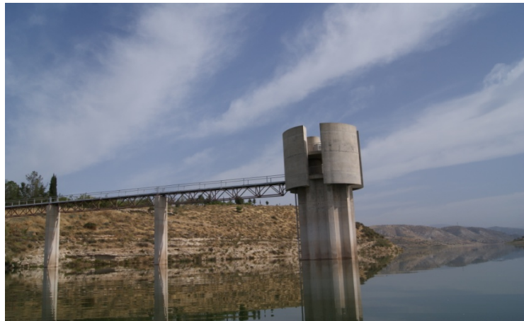
Figure 2. Picture of Asprokremmos Dam / Tower pumping station (Outlet Area)
