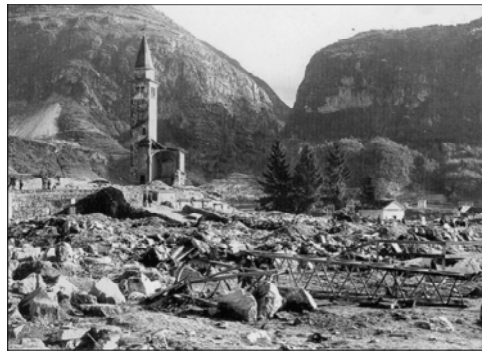
Figure 9. Pirago's bell tower: the only building left standing in the village after the transit of the wave (Zanfron, 2006).
