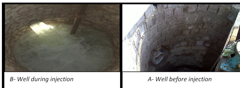
Figure 2. Recharge well- pumping before and during injection.
