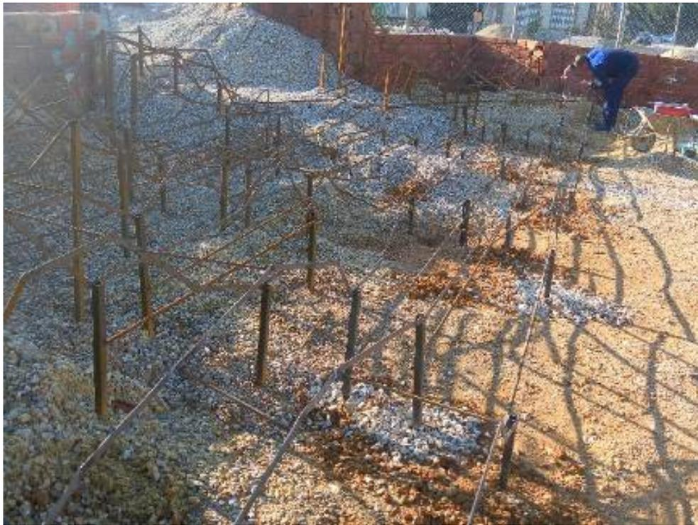
*Figure 4. Construction of downstream area.*
