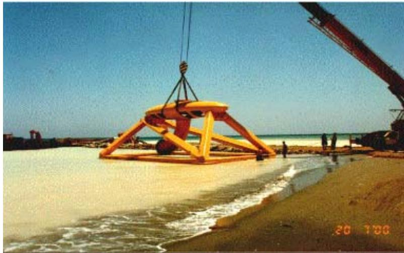
Figure 3. Larnaca desalination plant. Seawater intake structure (Courtesy of IDE-OCEANA).
